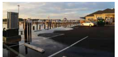
More frequent extreme high tides caused by sea level rise and subsidence inhibit access to the foot of High Street (left), prohibit boating visitors from tying up to the Wilmer Park bulkhead, and make for a soggy walk along the path (center). The “Walk In-Wade Out” still occasionally floods even after the Town raised the parking lot by two feet (right).
