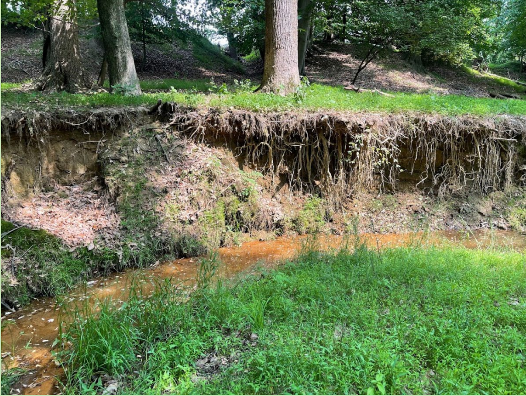
Unstable bank undercutting mature hardwood trees / major bank collapse
