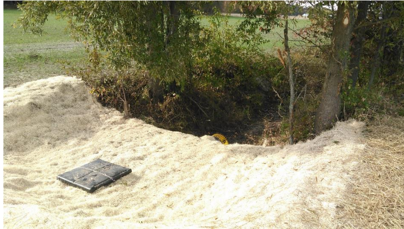
Figure 12. Structure for water control installed in a ditch to help control water level and increase nutrient removal within the ditch.
