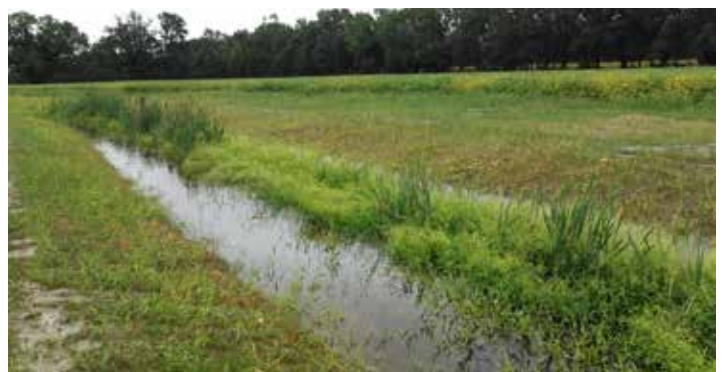
Drainage ditch management is one of the priority restoration practices we have identified to improve the quality of water running off fields. Left: a two-stage ditch under construction. Right: a completed two-stage ditch acts as a mini stream and floodplain, allowing for stormwater to slow down and percolate through plants and soil, removing nutrient and sediment pollution.
