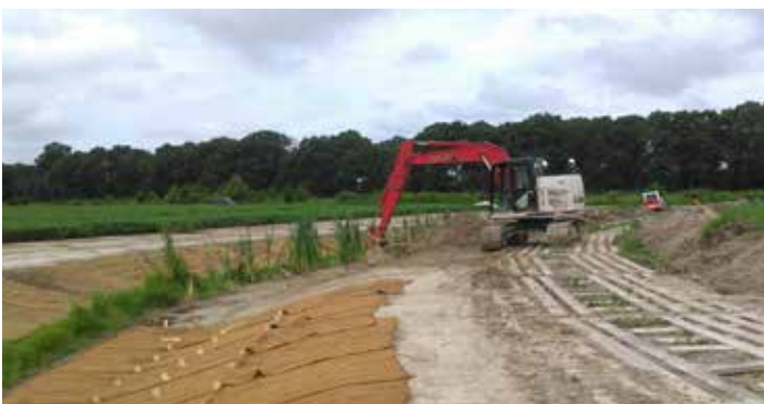
Drainage ditch management is one of the priority restoration practices we have identified to improve the quality of water running off fields. Left: a two-stage ditch under construction. Right: a completed two-stage ditch acts as a mini stream and floodplain, allowing for stormwater to slow down and percolate through plants and soil, removing nutrient and sediment pollution.
